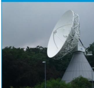
通信机器 Communication Equipment
